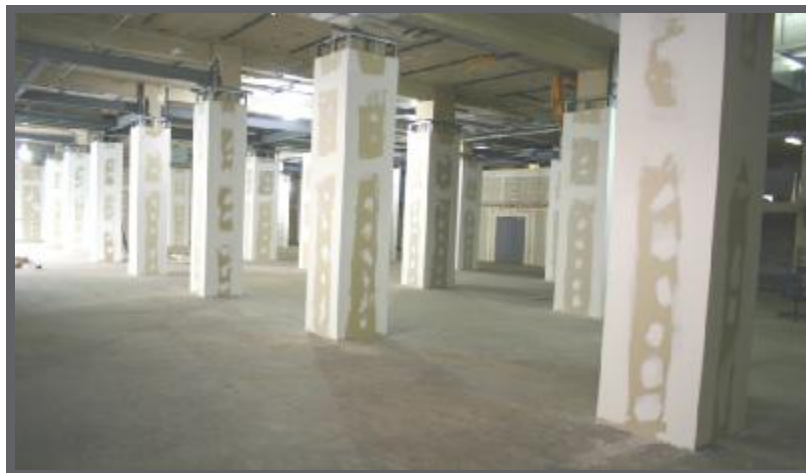
In-Progress Redevelopment 427 S. LaSalle Chicago, Illinois
